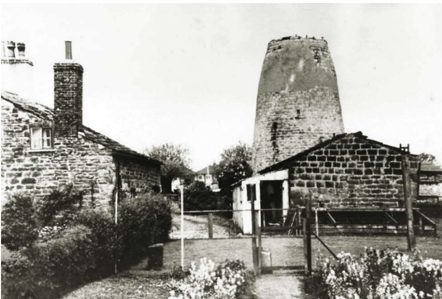
Left: This photograph was taken in 1963 It shows the derelict windmill and farm buildings, known as Windmill Farm or Betty Barker's Farm. The farmhouse and outbuildings were demolished in 1964 and the lead conical covering of the windmill tower was stripped sometime before. In 1973 the stone tower of the windmill was restored and incorporated into the new Windmill Hotel.
