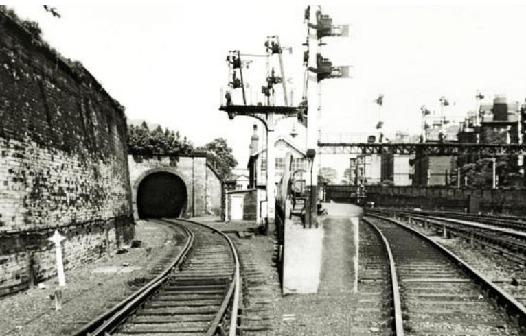
Left: This photograph was taken from the end of platform 1A at Scarborough Central Station showing the platform line on the right and the line through the Falsgrave Tunnel on the left. The tunnel carried only one track and was in use until 1965. The railway line has been lifted and tunnel entrance bricked up
