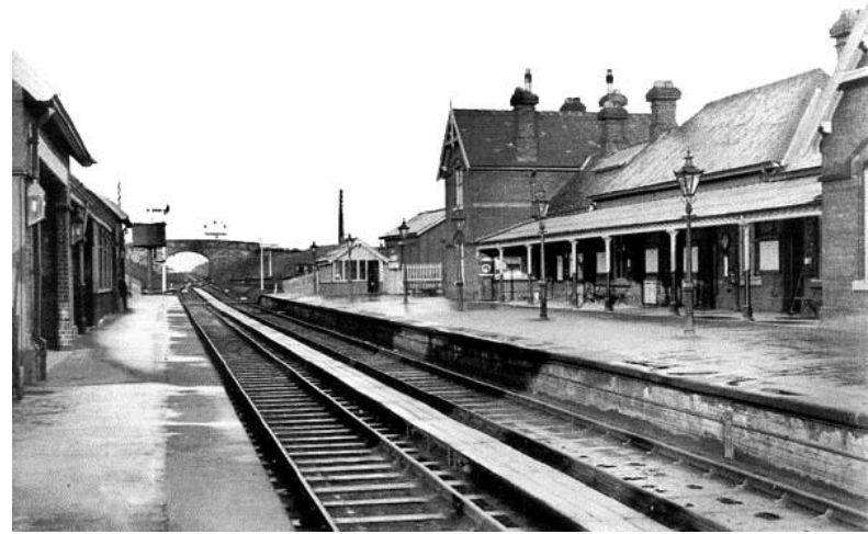
Right: This 1908 photograph shows Whitby West Cliff station looking north. The two-storey red brick station master's house can be seen on the 'up' platform next to the long single storey waiting room and booking office. Towards the end of the platform is the wooden signal box. On the opposite 'down' platform is the red brick waiting area and at the very end of the platform is a water tank. Further in the distance to the north end is a stone bridge over the railway line
