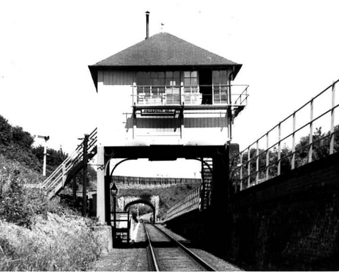
Left: The signal box at Prospect Hill Junction was a bridge type. This view is looking north towards West Cliff station. It commanded an excellent view of both the Whitby, Redcar and Middlesbrough Union Railway (WR&MUR) line below, and the Scarborough and Whitby line (S&WR) which ran above the retaining wall on the right. The pair of staircases allowed the signalman to reach platforms for the collecting and handing over of single line tokens. The signal box was destroyed by fire after the lines closed
