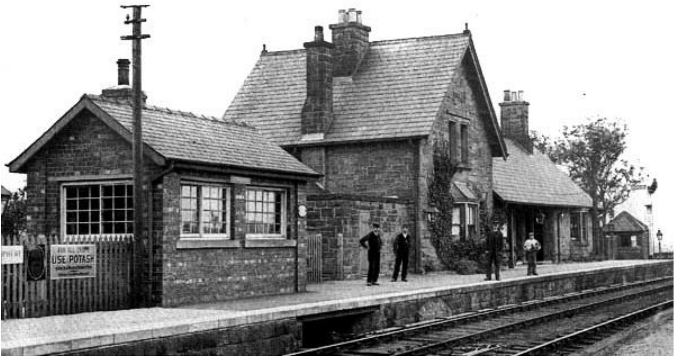
Above: Cloughton station in 1904 showing the two storey station master's house and to the right a single storey waiting room and offices
