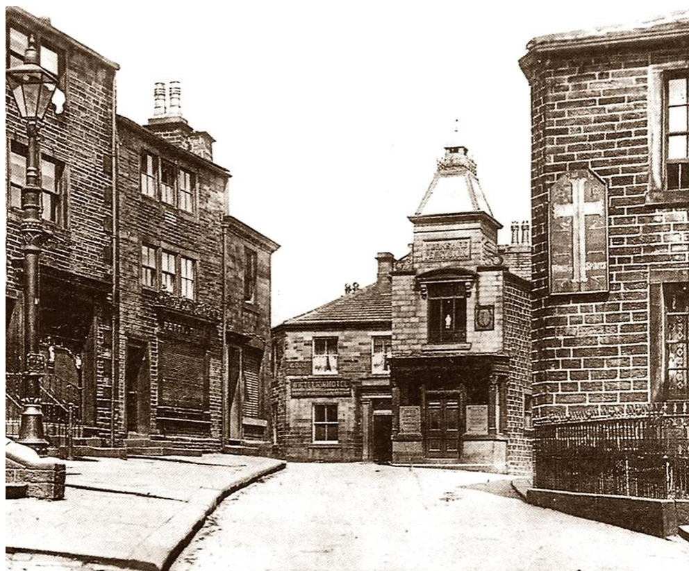
Right: This photograph was taken after a short tower and a pyramidal roof was added by the Yorkshire Penny Bank, the name YORKSHIRE PENNY BANK is carved in a rectangular block of stone.
