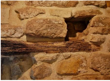
Left: Mediaeval oak lintel inside the building
