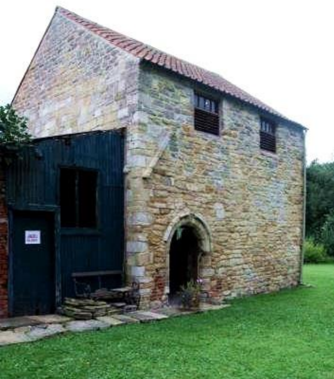
Left: The West Wall after restoration with a new roof and two new upper windows. The 12th century doorway has a new oak door
