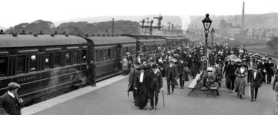
Left: A train arriving at Washbeck Excursion Station in 1913. Many passengers can be seen alighting and making their way out. The station was not renamed Scarborough Londesborough Road until 1933
