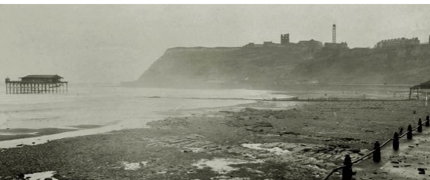
Left: This photo shows the extent of the storm damage to the North Pier in 1905. The whole structure was destroyed leaving the pier-head standing in isolation out at sea which was subsequently demolished. It also shows the Warwick Revolving Tower on the misty horizon.
