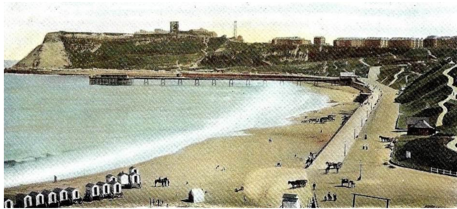
Right: This coloured postcard illustrates the Royal Albert Drive with bathing machines on the beach near the edge of the sea. The North Pier stretches out into the North Sea. On the horizon is the Warwick Revolving Tower with the ruins of Scarborough castle's keep on the left at the top of the rocky promontory.
