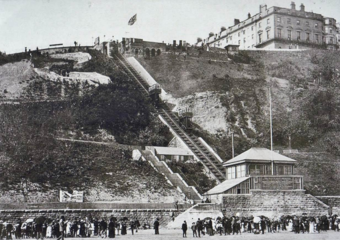
Left: The lower station building of the Scarborough South Cliff Railway in 1890. It is facing the sea, and has a tall hipped roof and there is a lower, lean-to extension with its famous roof sign. The lower part of the incline incorporates an arched tunnel to accommodate a pedestrian footpath from the gardens beneath the tracks which can be seen on the left side of the railway next to a small
